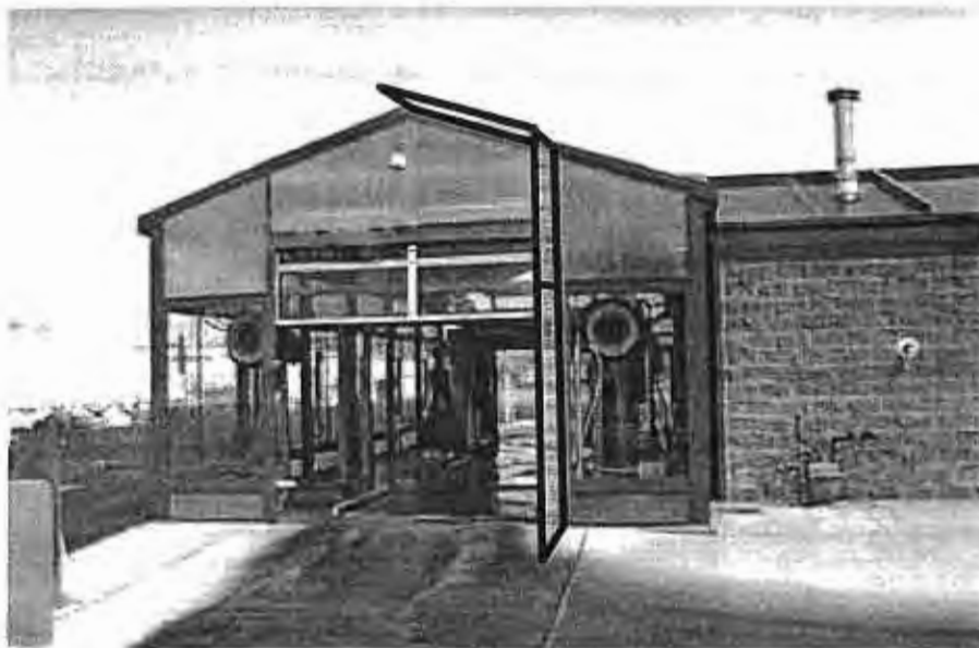
Figure 6. This figure evaluates the height of the 4-ft wall and shows that the car wash door opening contains line of sight (the door perimeter does not block it). Therefore, the roof edge extension shown in Figure 7 is added to the 4-ft-long barrier wall.
